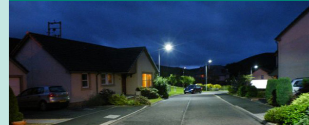
New LED Lighting
